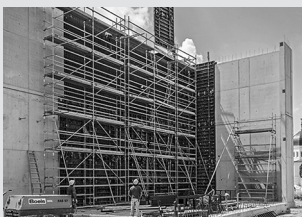
Working scaffolds for construction
