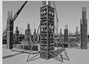
Column formwork
