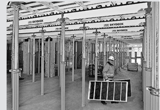
Slab formwork
