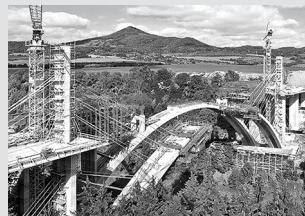
Bridge formwork
