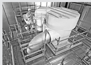
Working scaffolds industry
