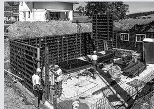
Wall formwork
