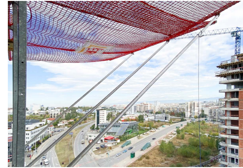
Catch Fans can be used as a safety net for people as well as for falling objects and small parts and, together with the PERI PROKIT Lateral Protection, offers an excellent safety solution for working at heights.
