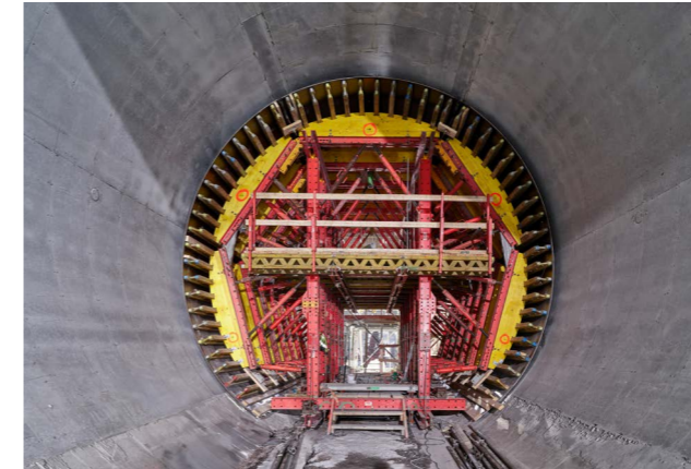
PERI's efficient tunnel formwork solution was instrumental in enabling the team to keep to the schedule during the freezing process.
