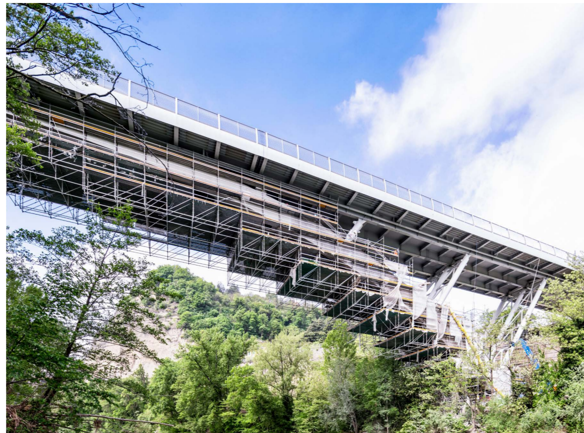
San Leonardo Bridge, Sasso Marconi, Italy
