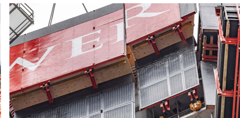
Premiere: The innovative MPS Pro Modular Protection Screen was used for the first time in the construction of the SkyTower.
