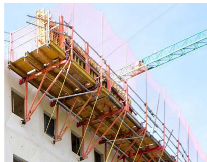
To construct the curved facade, engineers from PERI produced a customised formwork solution and combined it with the CB Climbing Formwork.
