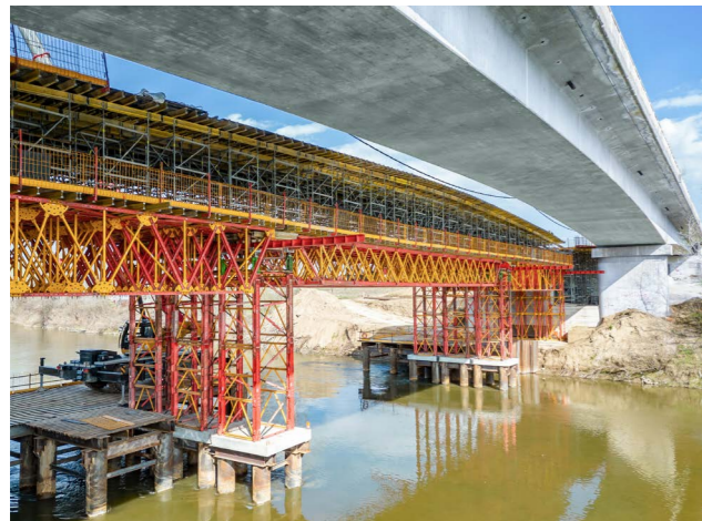
The coordinated delivery of the formwork and scaffolding solutions increased the cost-effectiveness of the project.
