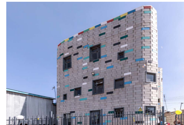
The Global One Primary School was built entirely from TwistBlocks, which were assembled without mortar.
