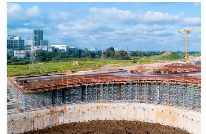
The complex shape of the bridge can be built without a special solution thanks to the flexibility of PERI Shoring Towers.
