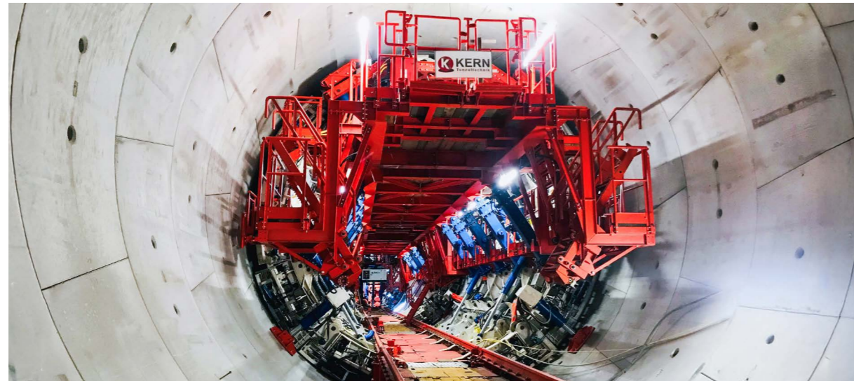
The merger with KERN Tunneltechnik SA enables us to offer our customers tunnelling solutions with an even greater degree of customisation.
