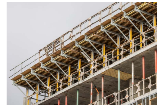
Image above: The combination of SKYTABLE and BR Shaft Platforms ensured an accelerated process, as the systems could already be installed on the next storey.
