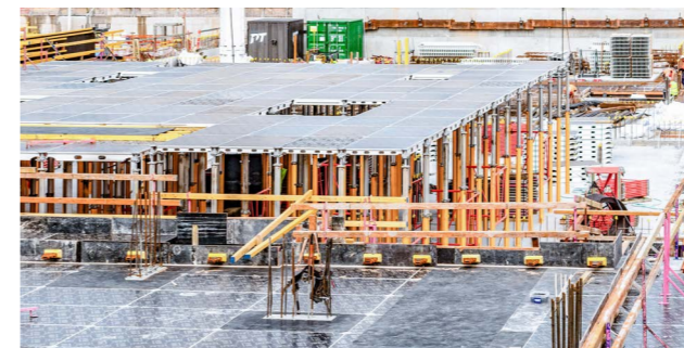
The PERI ALPHADECK formwork was used for 5,000 m 2 of formwork surface and impressed the customer in particular with its innovative drophead system for early stripping.
