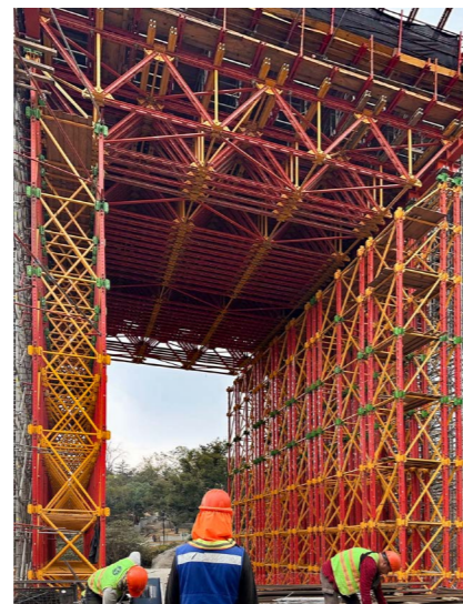
Due to the low weight of the ALPHAKIT Steel Components, the parts could be completely assembled by hand - without any lifting equipment.
