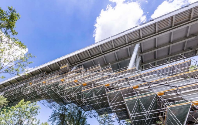
It was possible to scaffold the complex geometry of the bridge arch precisely using the PERI UP Modular Scaffold.
