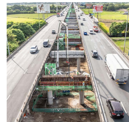
The customised PERI Solution facilitated rapid construction progress without interrupting traffic.
