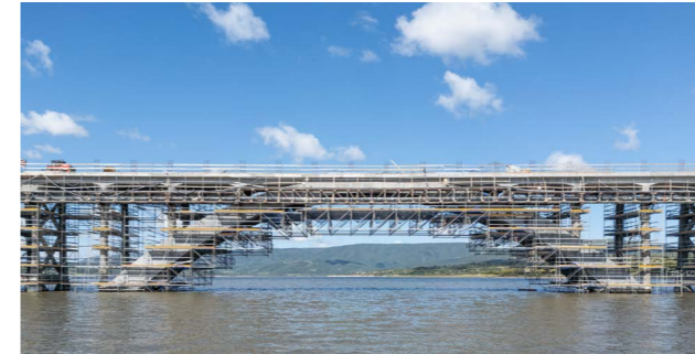
PERI’s adaptable working platforms provided safe access to the hard-to-reach arches and piers of the Diana Bridge.
