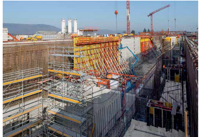
Comprehensive formwork solutions and a high degree of prefabrication also helped to deal with complex building geometries at a depth of 15 m - easily, accurately and on schedule.
