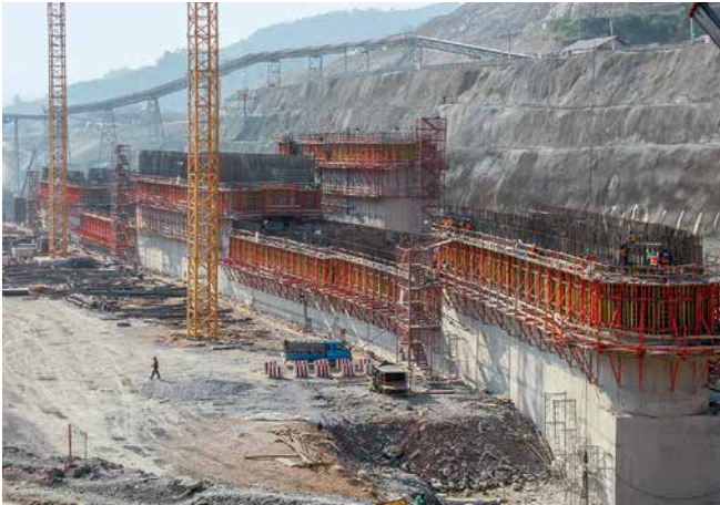
The high flexibility of the Climbing System SCS allowed an easy adaptation to suit all geometries in this dam project.
