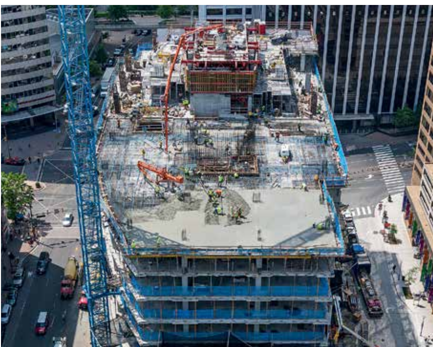
With the ACS Core 400, walls and slabs can also be concreted in one pour. For this, very large placing booms are used.
