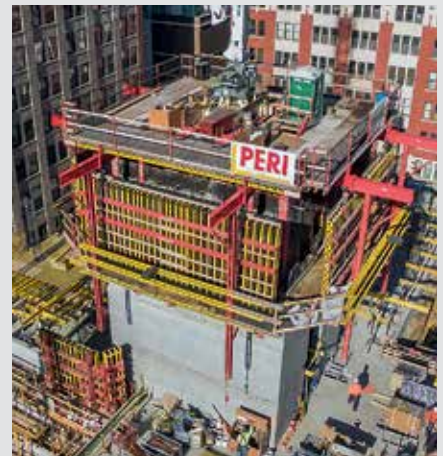
2016 CEB Tower at Rosslyn Central Place, Arlington, VA, USA (ACS Core 400)
