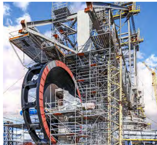
A total of 200 t of scaffolding material was required to scaffold the excavator, a piece of equipment that is over 190 m in length.
