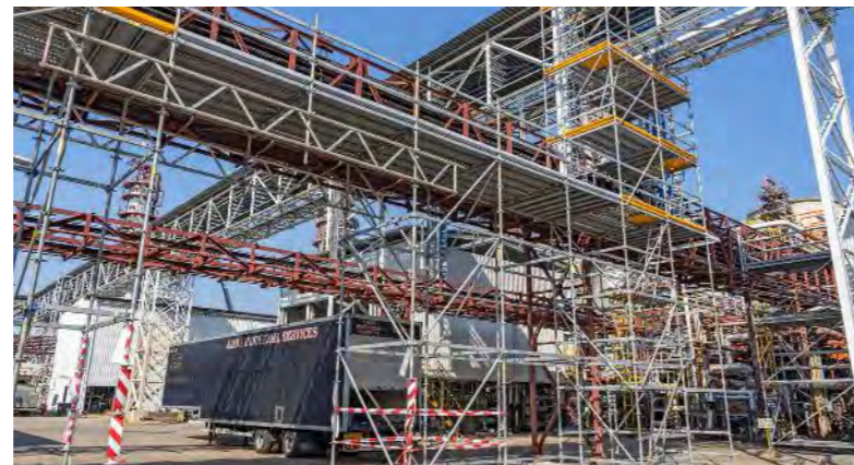
The gap-free decks with non-slip surfaces provided safe access even in confined spaces.
