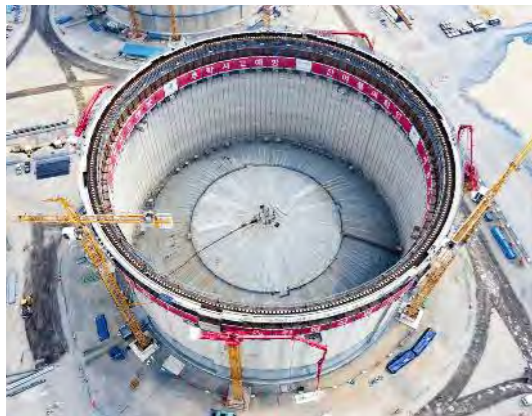
The use of advanced PERI Systems improved efficiency and safety on the construction site.
