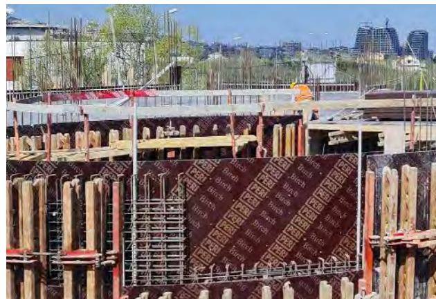
PERI Formwork Systems featuring PERI Birch Formwork Panels played a decisive role in the construction of the circular building sections.
