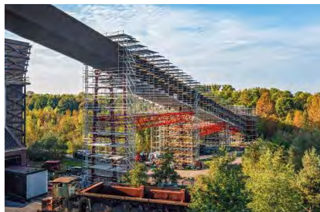
The 120-m long and 30-m high conveyor bridge was scaffolded cost-efficiently using two PERI Modular Systems – PERI UP and VARIOKIT.
