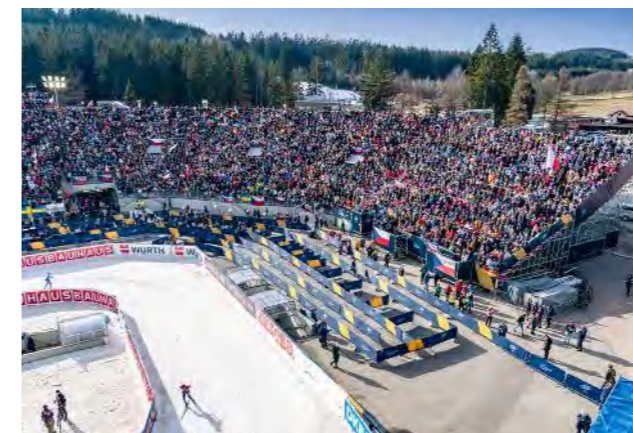
PERI UP Scaffolding and the PROKIT Lateral Protection System were used to expand the event infrastructure of the Vysočina Arena for the Biathlon World Championships.
