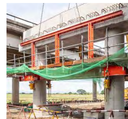
VPS paved the way for short concreting cycles and enabled the 250 cross girders to be completed on time.
