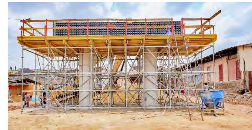
The small number of systems and components and their versatile deployment characteristics resulted in significant time and cost savings.
