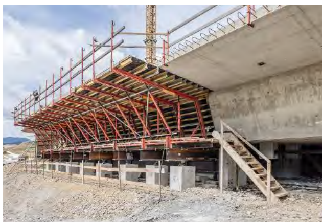
The VIL Incremental Launching Facility impressed with its high load-bearing capacity, leading to time and material savings.
