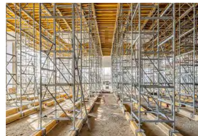
The use of PERI's compatible formwork and shoring systems enabled smooth integration and efficient execution.
