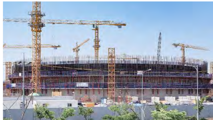
VARIO Girder Wall Formwork enables contractors to form walls in complex shapes and was therefore very well suited to the construction of the LNG tanks.
