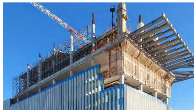
PERI helped the customer to keep to the tight schedule by shortening delivery and planning times for technical solutions.
