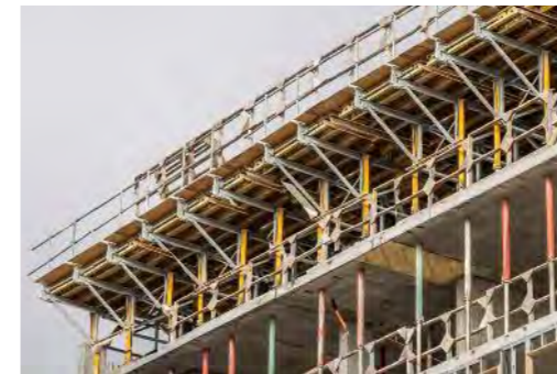
Image above: The combination of SKYTABLE and BR Shaft Platforms ensured an accelerated process, as the systems could already be installed on the next storey.
