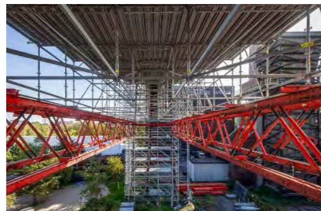
This PERI concept with wide-span VARIOKIT Truss Girders created space beneath the conveyor bridge and offered considerable savings potential.
