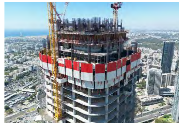
The use of self-climbing systems has reduced crane operating time and increased efficiency.
