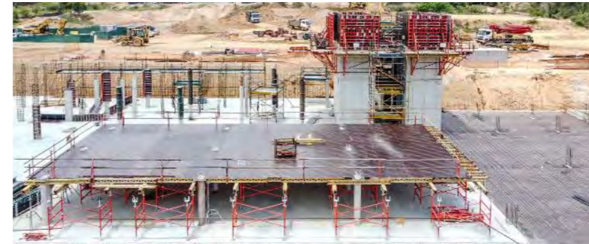
Pre-assembled slab tables were used to ensure efficient production of the slabs, thus increasing productivity on the construction site.
