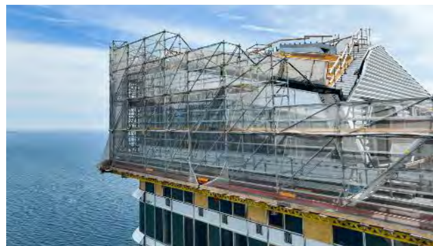
A fine-meshed net was installed at a height of around 140 metres to increase safety.
