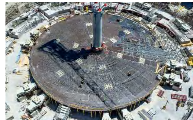
The base in the centre of the ELT was built quickly and flexibly with the aid of MULTIFLEX Girder Slab Formwork.
