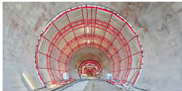
To ensure a high-quality concrete result, the curing gantries controlled the temperature and humidity along the tunnel formwork.
