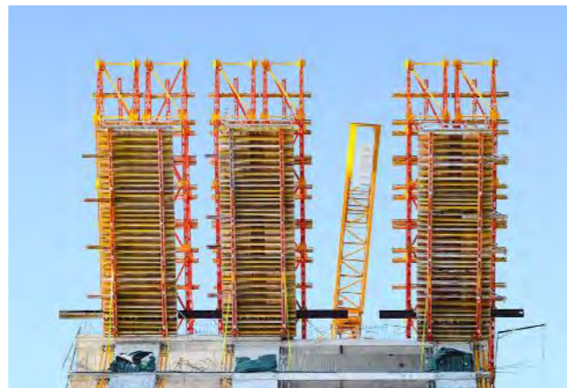
With a cleverly coordinated step-by-step plan, PERI made it possible to construct the sophisticated cantilevered balconies without any issues.
