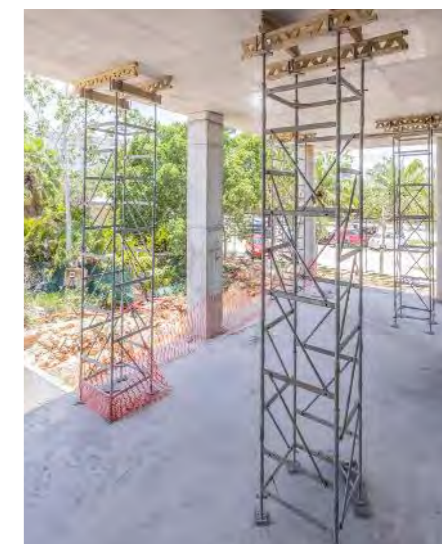
The ST 100 System was assembled using plug-in connections. As such, there was no need for connecting bolts or other parts that could easily go missing on the construction site.
