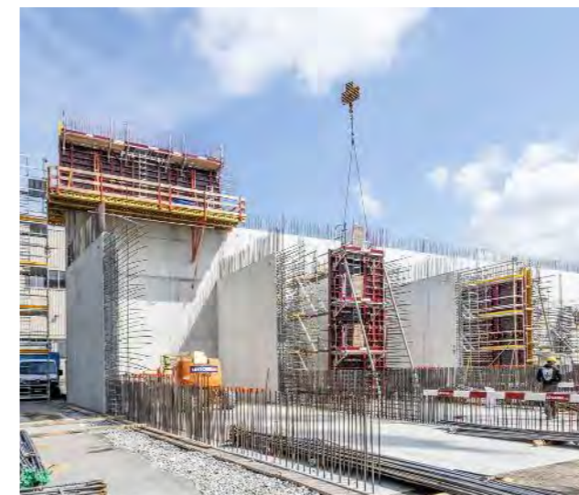
Construction progress was accelerated by the fact that many of the PERI Systems used could be moved by crane.
