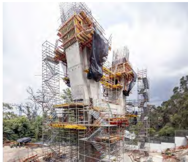
A combination of coordinated PERI Systems accelerated the construction work on the Manantial Bridge.
