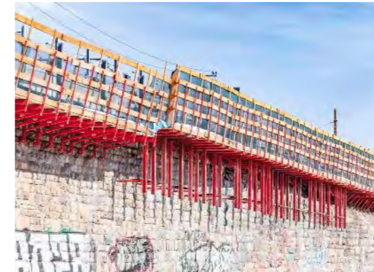
Having the formwork unit separate from the work platform was a particular advantage, as it meant that the deck was closed at all times.
