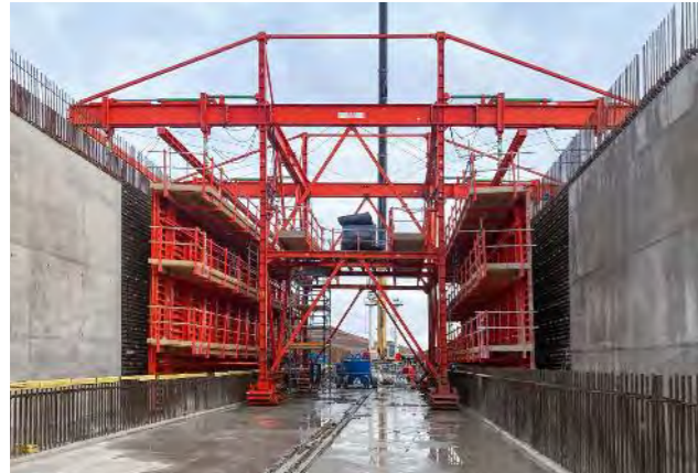
The customised formwork carriages consisted of a combination of special parts and VARIOKIT Standard Components and made a decisive contribution to efficient use.
