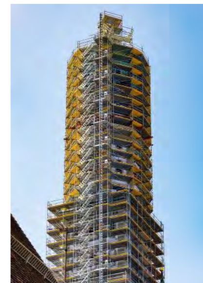
The transition from a square to octagonal cross-section halfway up the tower presented engineers with a unique challenge that was ultimately solved with the use of a PERI UP Scaffolding Kit.
