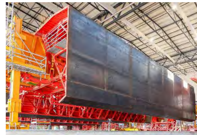
The special-purpose formwork designed by PERI's engineers is a key part of the production process for the 79 standard tunnel elements.
