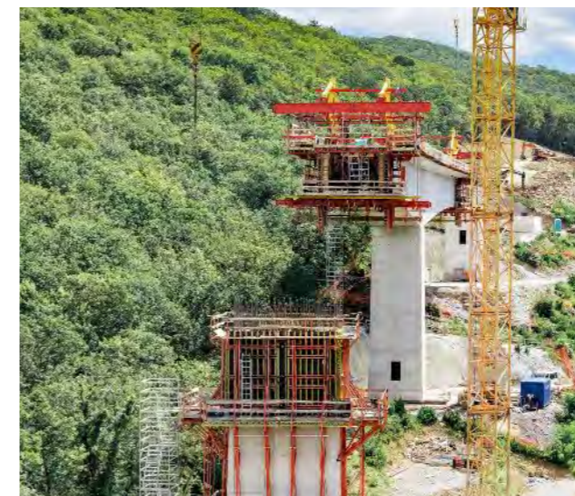
Thanks to the VBC System, it was possible to make rapid construction progress despite the challenging environment.
