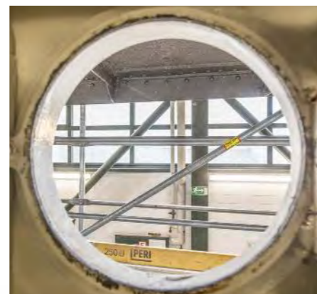
PERI delivered an efficient scaffolding solution to meet the specific requirements of this unique project.
