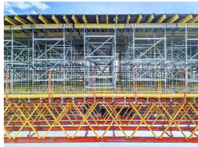
A well-thought-out combination of PERI System Solutions made it possible to construct the spans efficiently.
