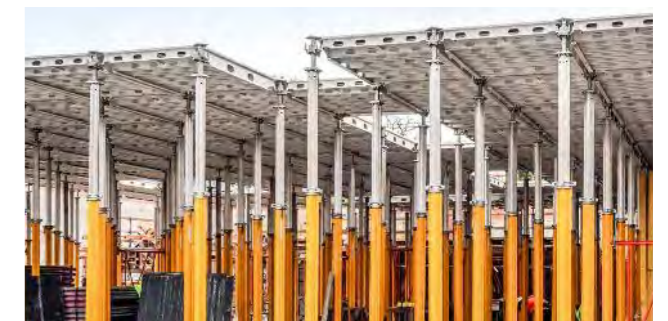
The combined use of ALPHADECK and MULTIPROP saved the customer time and labour.
