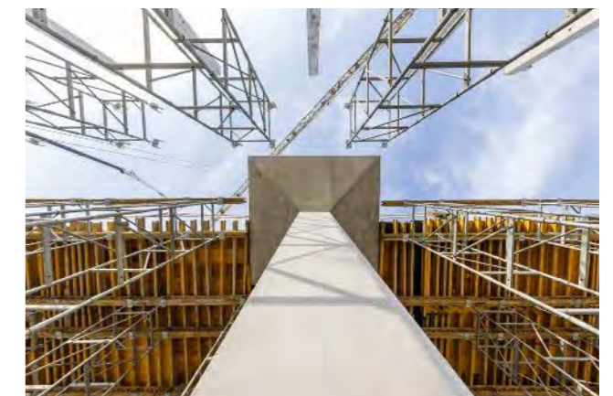
A combination of several formwork systems provided the central building block for the prefabricated columns with bases in the second and third sections of the hall.
