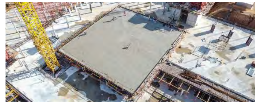
The compatibility of the PERI Systems contributed to the fact that the time and cost framework required for the construction site could be adhered to.
