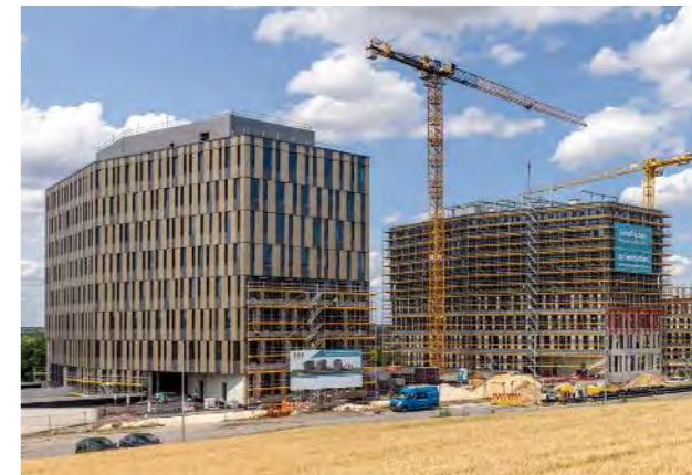
Approximately 5,000 m 2 of PERI UP Scaffolding was used for each of the individual office towers, which grew upwards during construction and were dismantled again during the installation of the facade.
