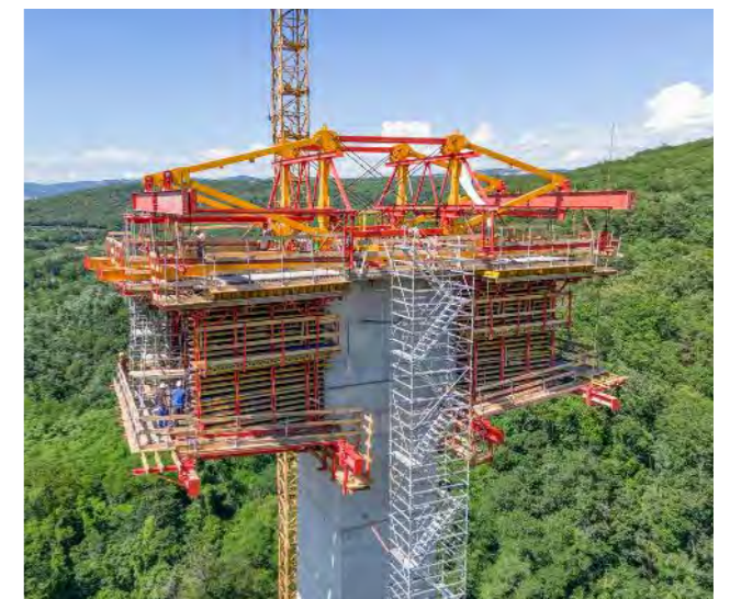
Rentable system parts ensured cost security and optimised use of materials.
