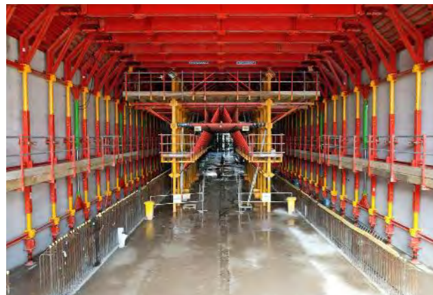
The formwork carriages helped to reduce cycle times by up to 80% and keep crane operating times short.
