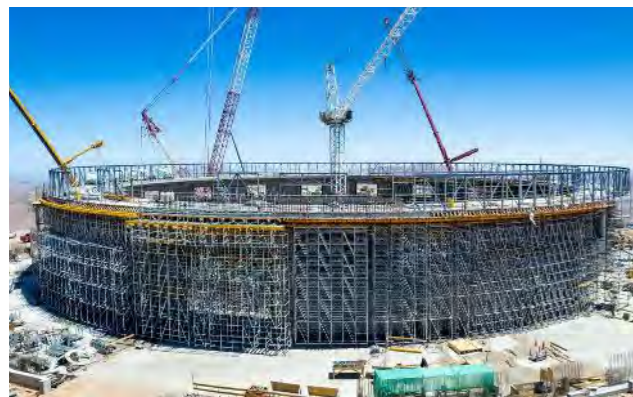
By combining the ST 100 Stacking Towers with components from the PERI UP Scaffolding Kit, access to the platform could be enabled.
