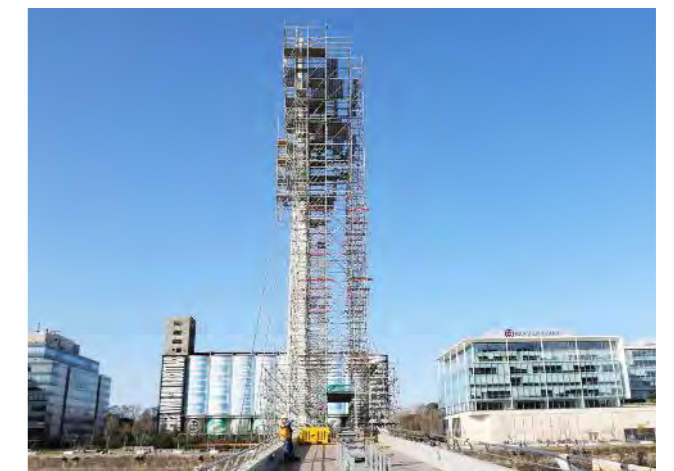
The scaffold used for renovating the mast of the Puente de la Mujer was 40-m high and solved the challenge posed by the low load limit of the pedestrian bridge.
