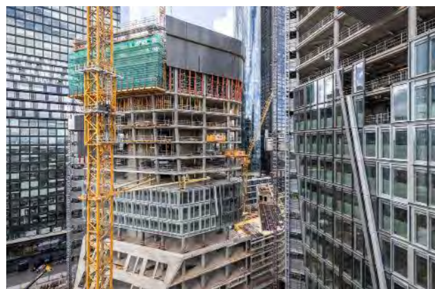
PERI Climbing Protection Panels were used to completely enclose the leading edges of the towers' upper floors.
