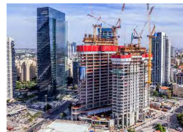
Both the office and residential towers were erected quickly and efficiently using a climbing system.
