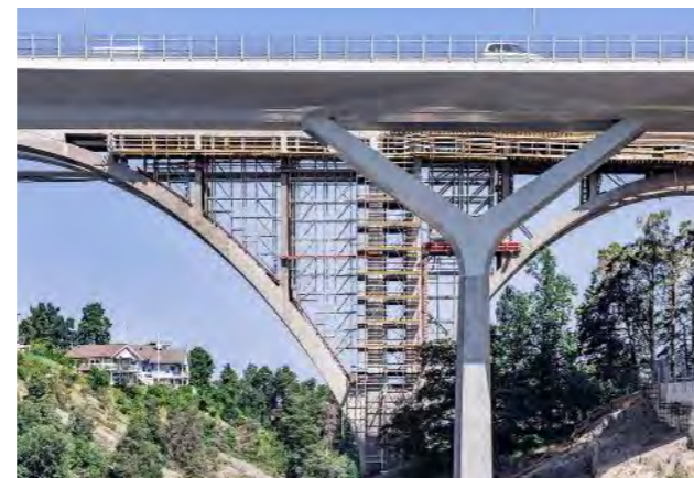
The arch of the bridge was built at a height of 32 m. PERI provided project-specific solutions and technical expertise.
