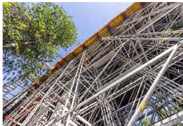
The combination of scaffolding, formwork and climbing systems made for a stable overall solution.
