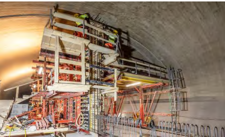
Technically sophisticated engineering solutions from a system combination of VARIOKIT and PERI UP contributed to the successful construction of the Brenner Base Tunnel.
