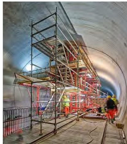
A high level of safety was made possible by the PERI UP Reinforcement Scaffolds when working on the formwork. These are ideal for construction site activities such as reinforcement, forming and concreting.
