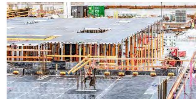
The PERI ALPHADECK formwork was used for 5,000 m 2 of formwork surface and impressed the customer in particular with its innovative drophead system for early stripping.
