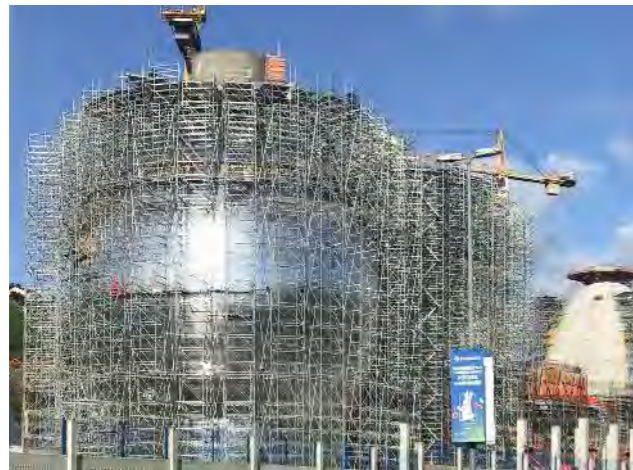
The eggshaped digesters placed special demands on the formwork and scaffolding technology, which PERI was able to provide with solutions.
