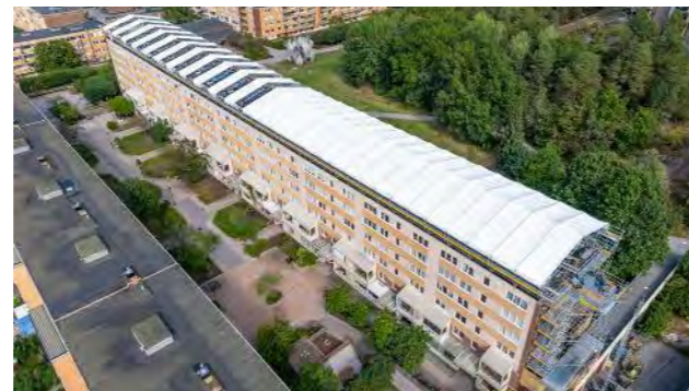
The logistics of transporting the work materials upwards was solved by using a working platform made of system components and a material lift.
