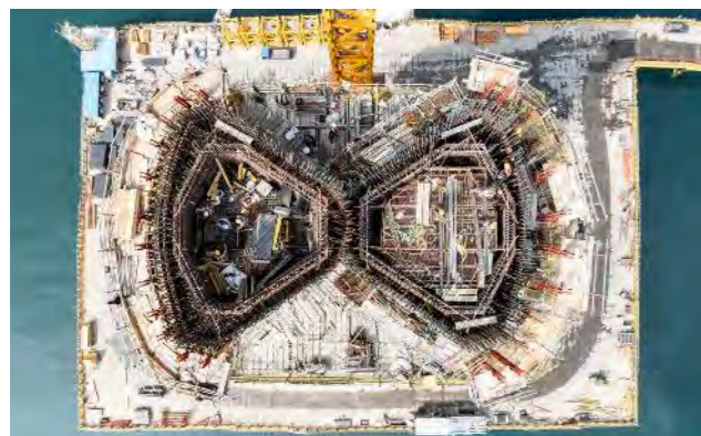
The cross-section of the pylon changes from convex to concave. The engineers from PERI therefore developed a customised formwork solution for each section.
